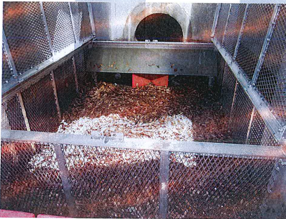
Nutrient Separating Baffle Box with trash / debris collected inside the screening system basket.
