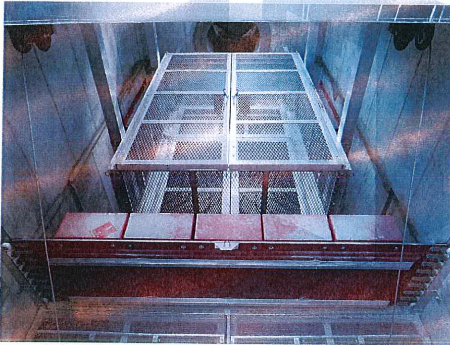
View of Nutrient Separating Baffle Box and SkimBoss Upflow Filter
