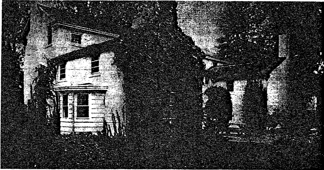
Another View of Barry — Mahan Home
